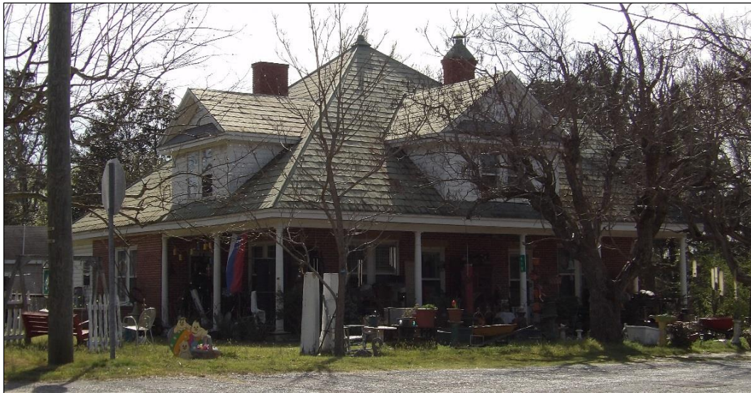
Photo 12: Northeast Oblique of the House at 610 Parks Street in Carthage.
