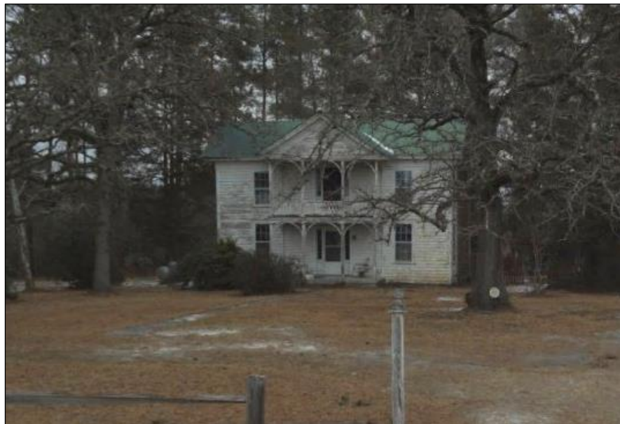
Photo 24: Southwest Elevation of the Ferguson-McDougald House (MR0554). 103
