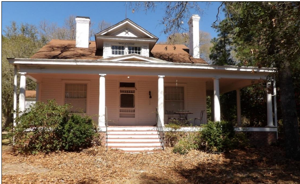
Photo 1: Dwelling, Southeast Elevation.
