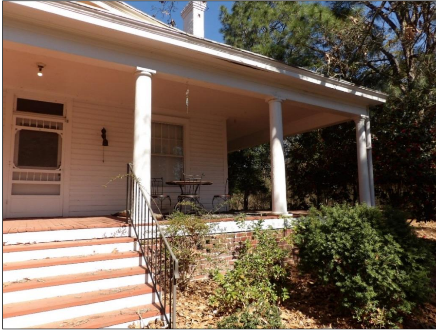
Photo 5: Detail of East Half of Porch, Looking North.
