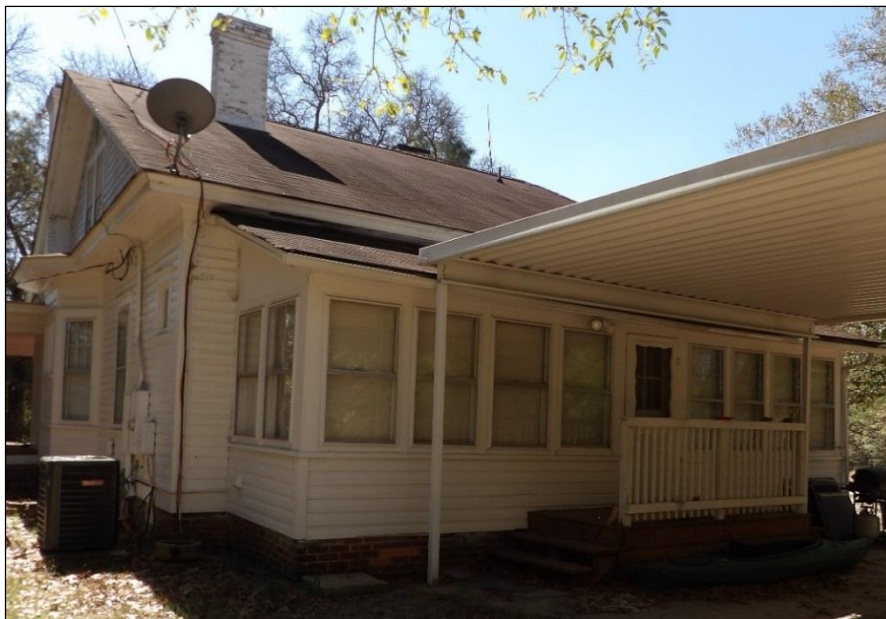
Photo 6: Addition on Northwest Elevation and Carport.
