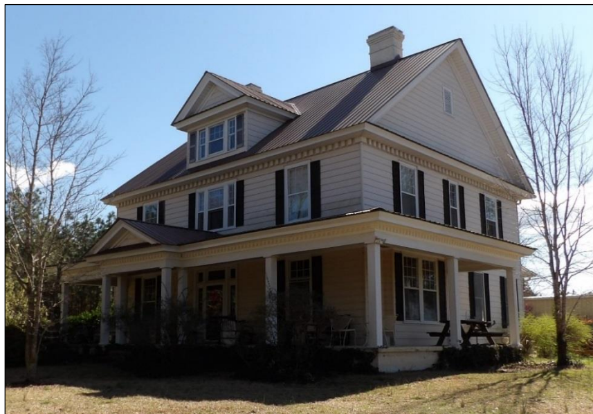
Photo 13: Dwelling, West Oblique.
