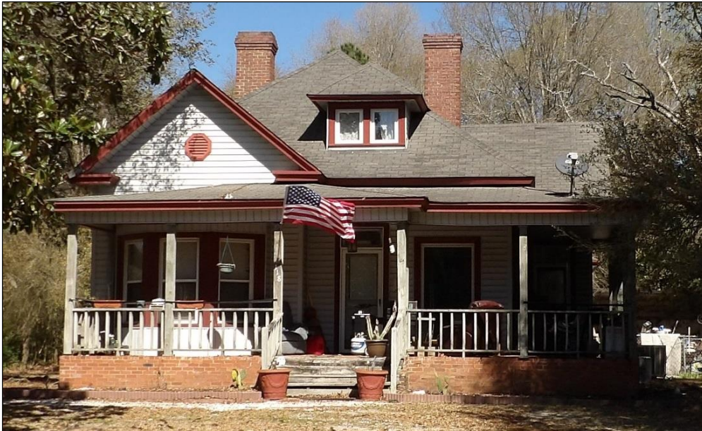
Photo 11: South Elevation of House at 2281 NC 73 Highway.
