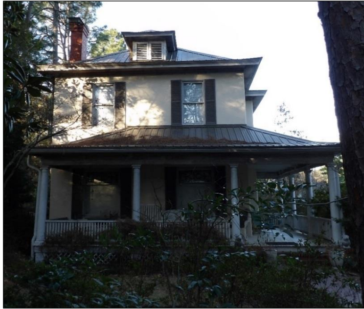
Photo 23: Stroud-Osbourne House (MR0353), Northeast Elevation.
