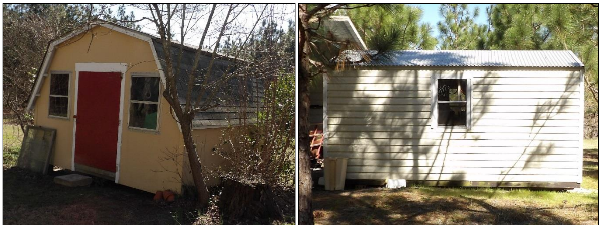
Photo 21: Shed, Looking Southeast (left); Prefabricated Shed, Looking North (right).
