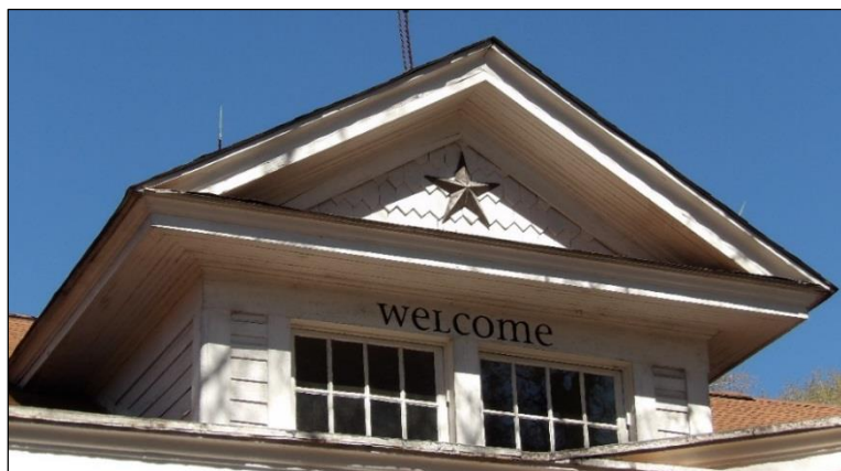
Photo 3: Dormer on Southwest Elevation, Looking North.
