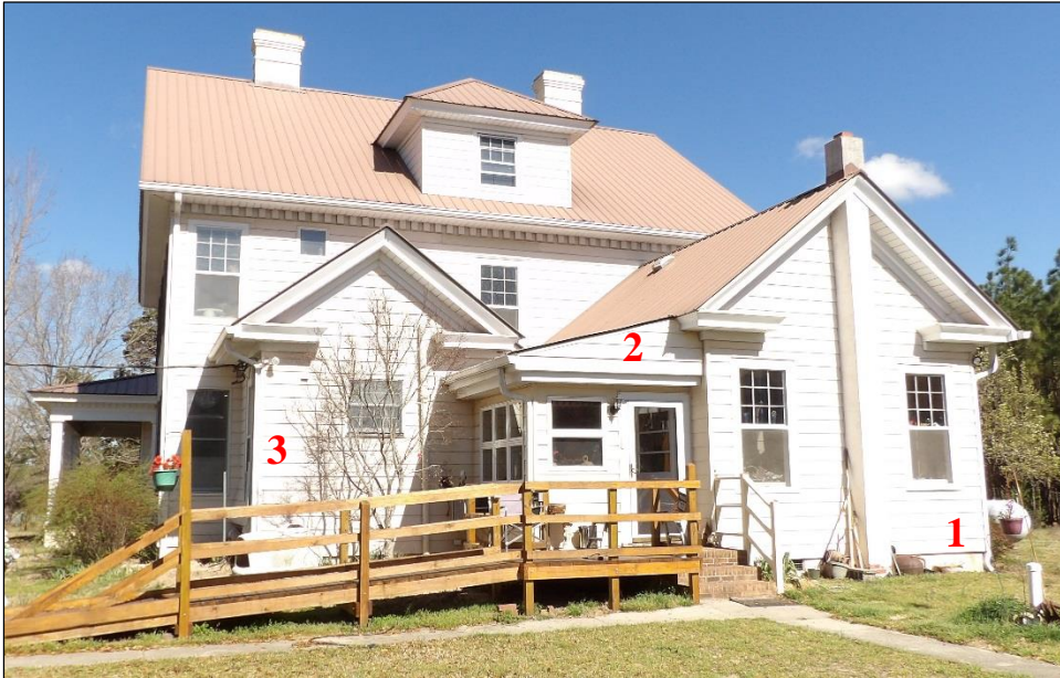
Photo 18: View of Additions on the Southeast Elevation, Looking North.
