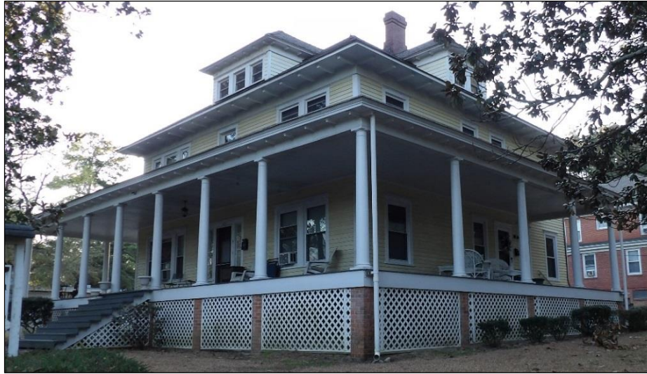
Photo 22: Northwest Oblique of the Lewis-Pennsylvania House (MR0378).
