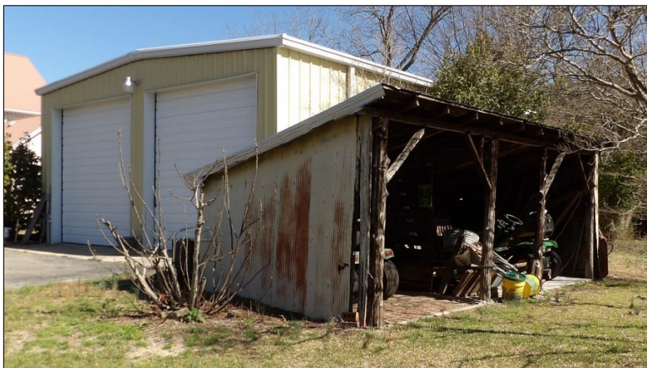
Photo 20: Garage and Machine Shed, Looking Northeast.
