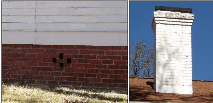
Photo 2: Foundation, Southwest Elevation (left); South Chimney, Looking Northeast (right).
