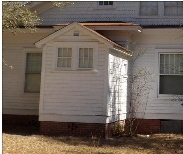
Photo 7: Gabled Addition on Southwest Elevation.
