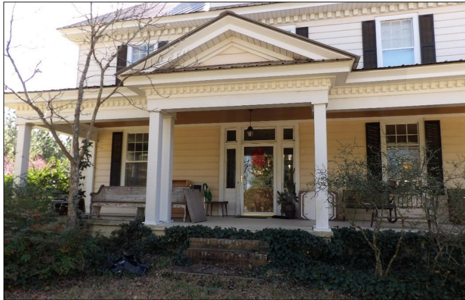
Photo 17: View of Primary Entrance of the Dwelling on the Northwest Elevation.
